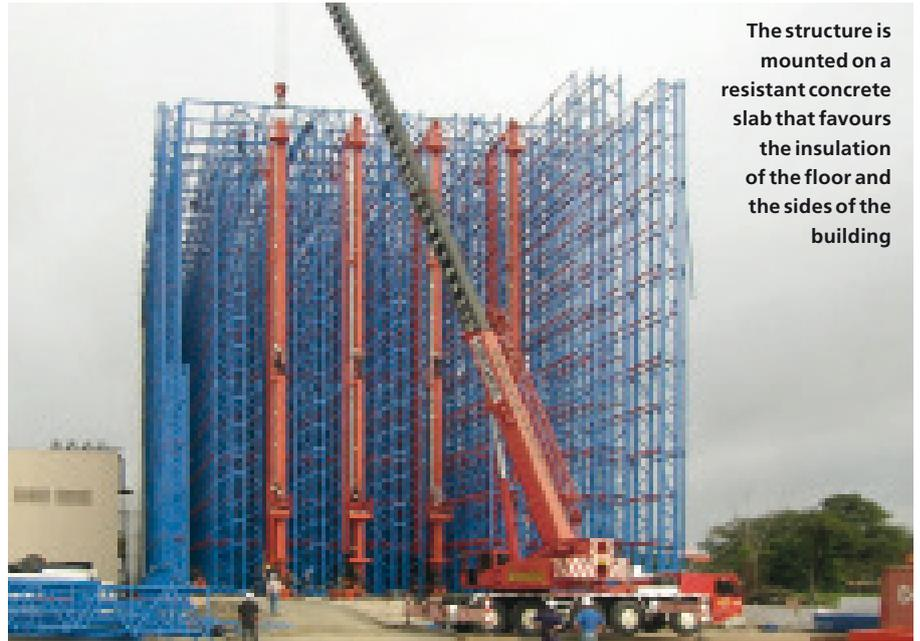
The structure is mounted on a resistant concrete slab that favours the insulation of the floor and the sides of the building
