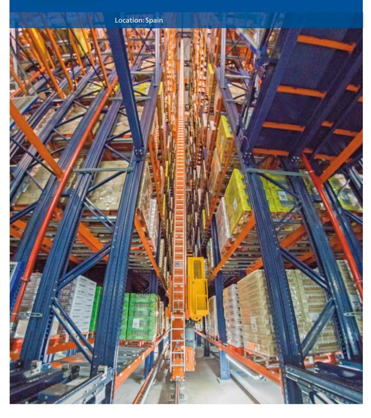
Mecalux builds DAFSA an automated clad-rack warehouse, in the scenic countryside near Valencia, whose outer finish was carefully made to be environmentally friendly. The new warehouse, with a capacity for more than 23,000 pallets, is integrated with production outputs via a twolevel overpass. Mecalux's Easy WMS (warehouse management software) was supplied to control all warehouse processes.
