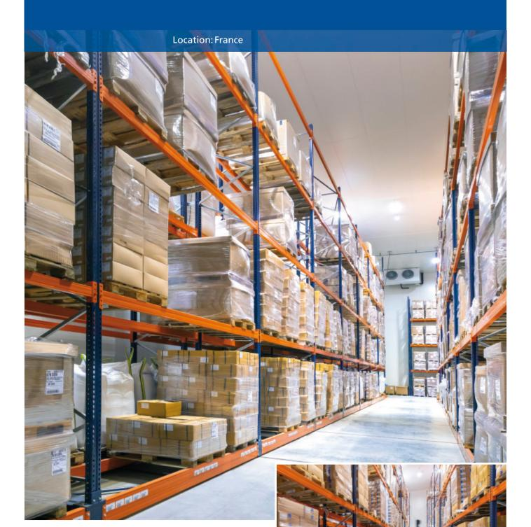
The Sabarot frozen-storage chamber in Chaspuzac (France) has 9.5 m high Movirack mobile pallet racks by Mecalux. This solution leverages all available surface area to achieve higher storage capacity and reduces power consumption to chill the installation. In total, 1,816 pallets can be deposited here filled with finished products.
